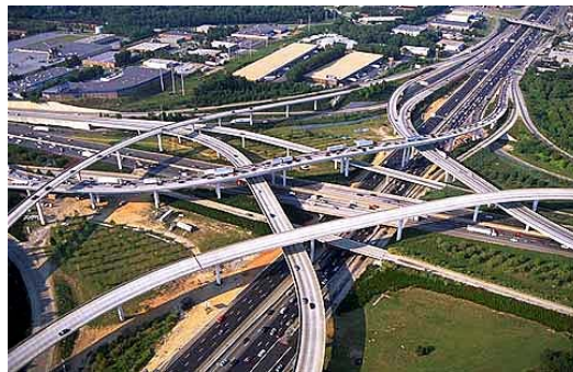
The District-wide WMP suggests that the GDOT comply with the stormwater management criteria outlined in the Georgia Stormwater Management Manual to control impacts of runoff from roadways.
